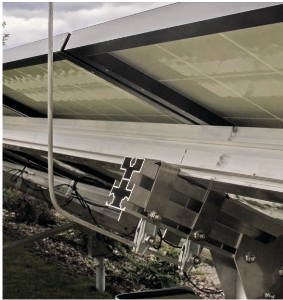
Figure 2 Lightning protection by means of DEHNiso spacers
