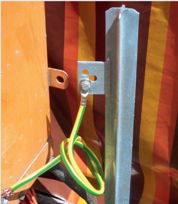
Profiled earth rods for the installation of earth-termination systems e.g. for antennas or construction site distribution boards
