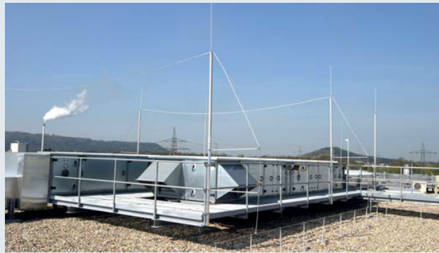
Isolated air-termination system DEHNiso Combi
