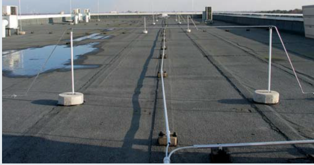
Elevated air-termination system with spacers and concrete bases in the range of the electrical installation on the roof
