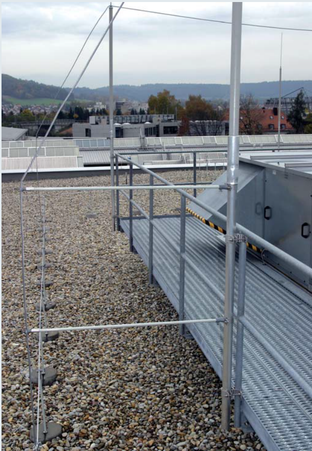
Spacers at the supporting tube
