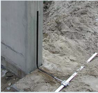
Earth entry rods to connect down conductors to the earth-termination system
