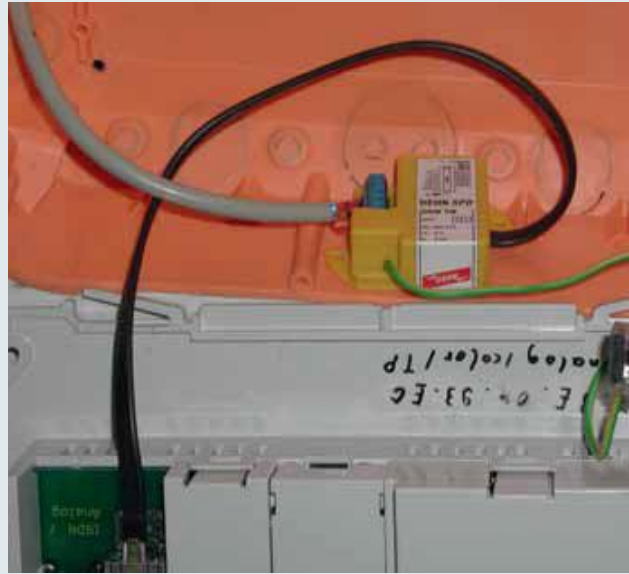
Flush-mounted surge arrester used in LAN interfaces
