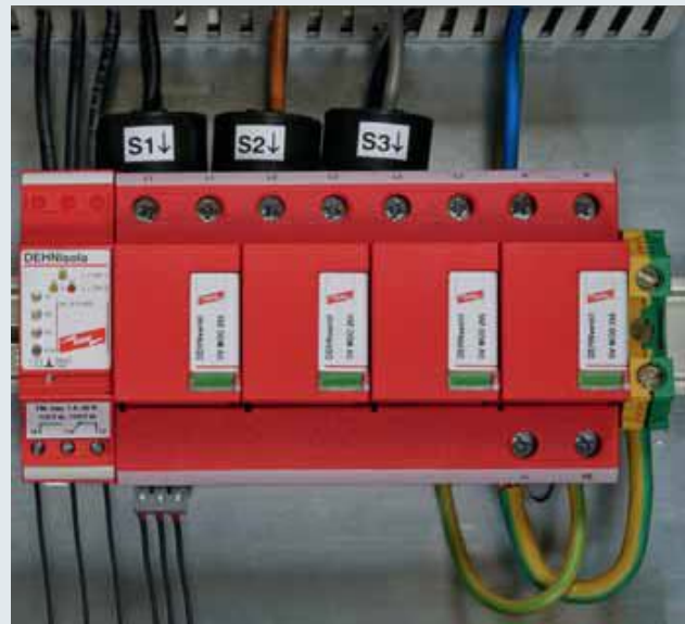
The DEHNisola monitoring device continuously monitors the function of installed lightning current and surge arresters
