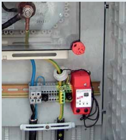
Counter with integrated battery supply (9 V) and battery charge control. Indication via two-digit LCD with setting and resetting buttons.
