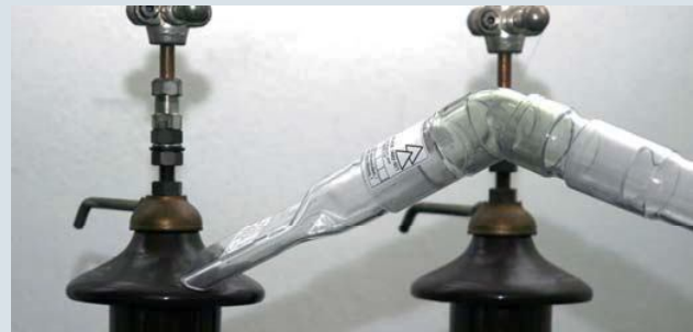
Cleaning an insulator with a flat cleaning head and 135° angled intake tube
