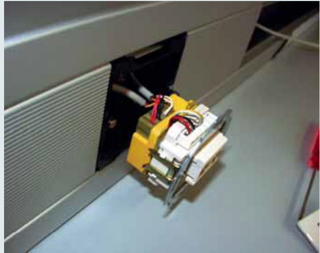
Surge arrester for protecting telecommunications equipment and installation into flush-type boxes or small-sized distribution boards. Plug-in terminals on the input side.
