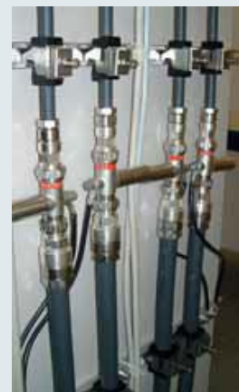
Application of quarter-wave arresters
