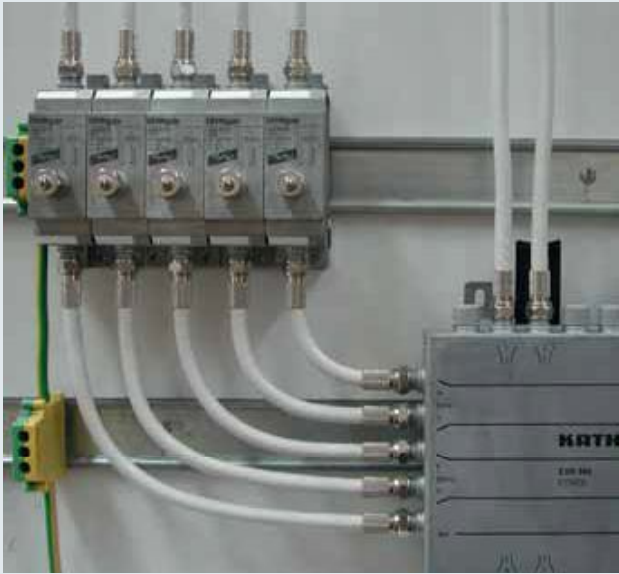
Lightning current / surge arrester designed as a cable adapter for protecting coaxial systems such as CCTV, mobile radio stations and antenna systems from potential damage.
