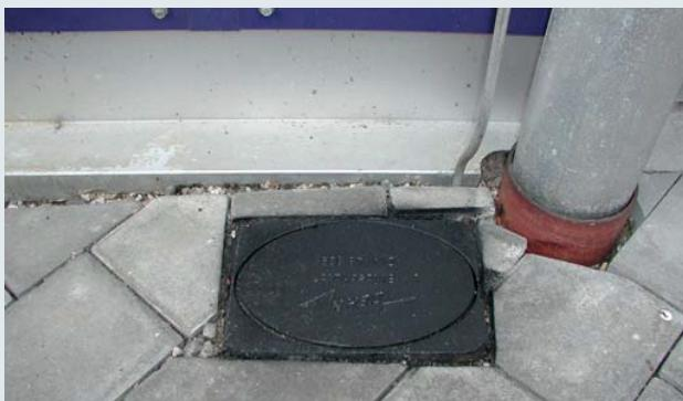
Test joint boxes for underfloor mounting, to disconnect the down conductor from the earth-termination system for measuring purposes
