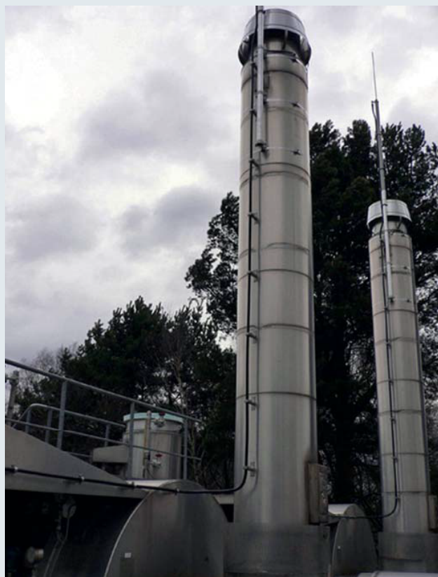
HVI conductor installed in Ex zone 2
