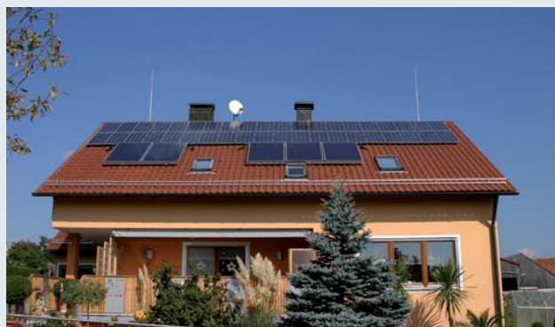
Isolated air-termination system – all roof-mounted structures such as solar thermal, PV and exhaust systems incl. the parabolic antenna in the protective area
