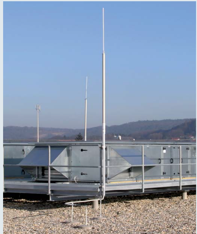
Isolated air-termination system for recooling plant with HVI conductor grey in a supporting tube
