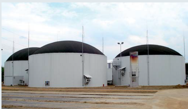
Biogas/natural gas plant Kerpen, Germany Protection of the fermenters – air-termination masts with HVI Conductors
