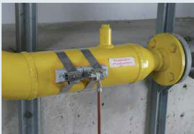
Pipe clamp for electrical contacting of pipes in explosion-hazard areas for implementing of lightning equipotential bonding according to EN 62305-3 (DIN VDE 0185-305-3)
